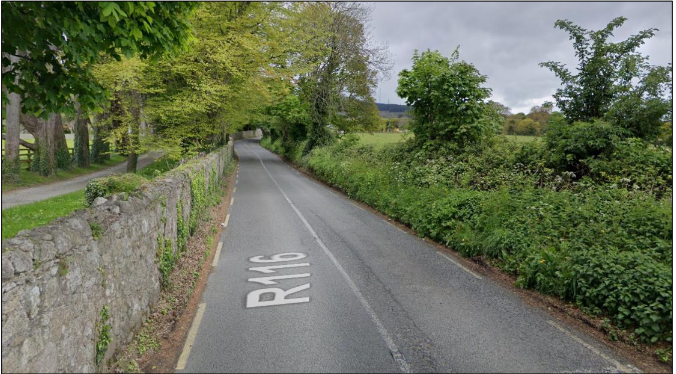
Figure 3-9 - Ballybetagh Road R116 Typical Road Section (source: google maps)
